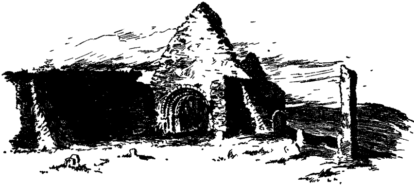
REMAINS OF OLD CHURCH AND ROUND TOWER AT KILCULLEN
